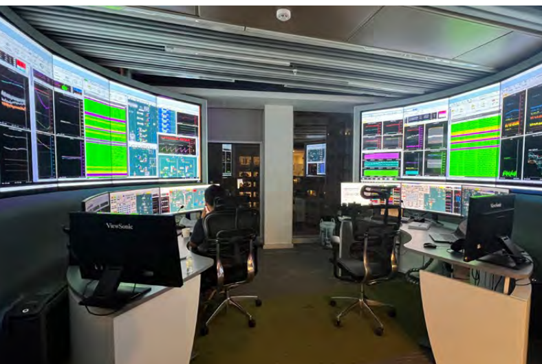
Remote Operation Control Center
