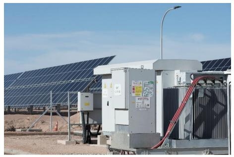
→ Location: Located in Region of Antofagasta, Chile, at 2,800 m altitude. → Installed Capacity: 81 MW // 210,672 solar panels + 80 MW \* 3h (BESS). Description: AES Solar IIA comprises 148,176 bifacial solar panels of 380Wp and 62,496 bifacial panels of 385Wp, in addition to 80 MW x 3 hours battery storage systems. → Total Annual storage estimated: 89 Gwh
